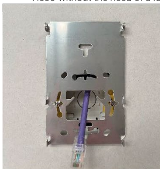
The Mounting Plate is screwed to the flush mounted back box & an RJ45 plug is fitted to the cable end
