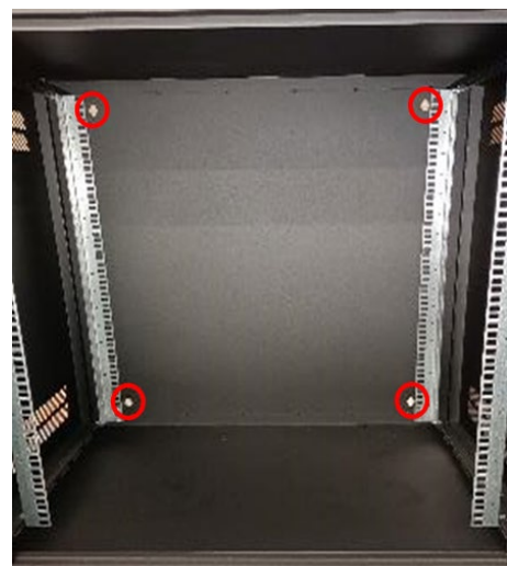
Fixing points viewed from inside the cabinet
